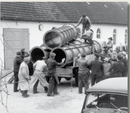
The loading of concrete pipe moulds on a truck in 1940 required much man power.
