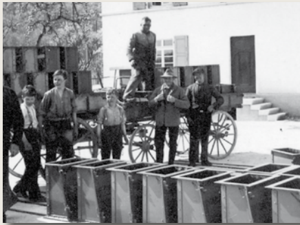
Concrete moulds are picked up with horse-drawn vehicle about 1907
