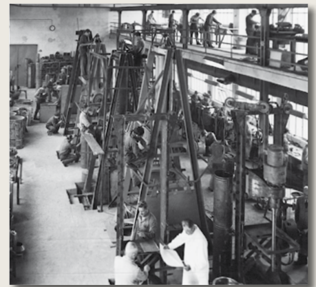
Production hall Ettlingen approx. 1938
