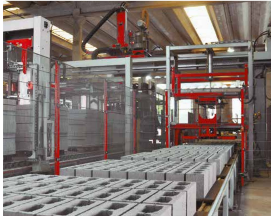
Dry side with hollow blocks
