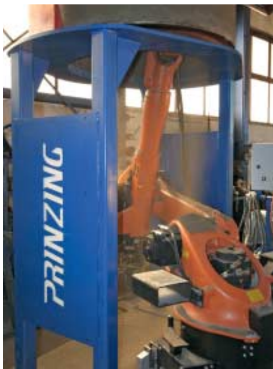
Fig. 4 Milling of drains on the milling unit.
